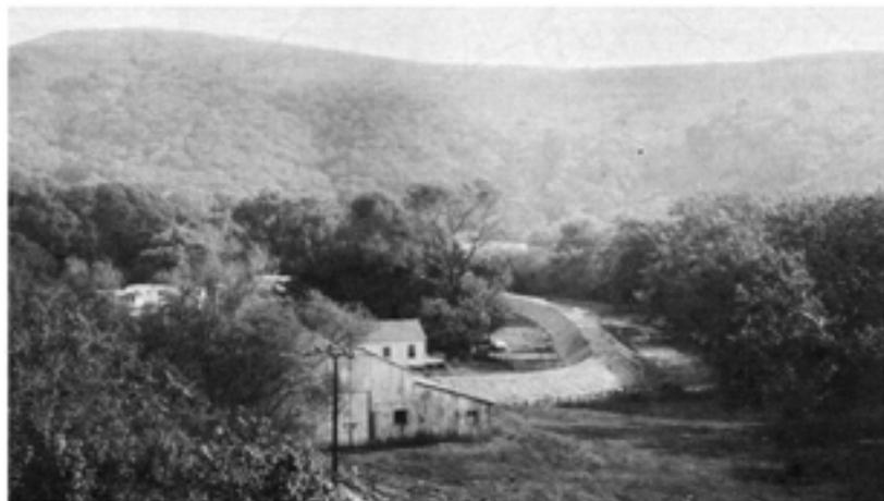
Photo 3. Dikes around structures near mouth of lower Big Sur River. Dikes were constructed to provide protection from floodwaters.
