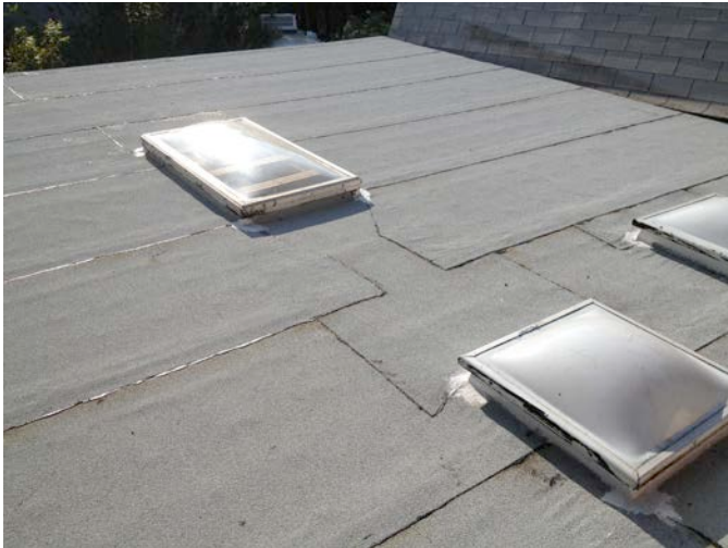
New roof on the Little House.
