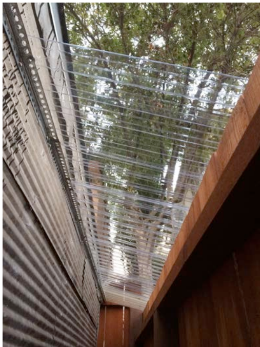
New fence and tool-shed cover around the Little House.
