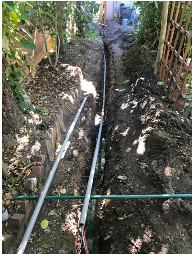
Before putting down new stone, I extended a 20-amp circuit underground adding outlets for the fountain and the barbeque rotisserie.
