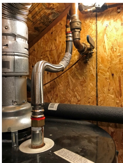
So it now has two new lines with stainless-steel wire mesh.
