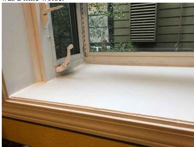
I cut a template then matched it to a new base, sealed it, and painted.
