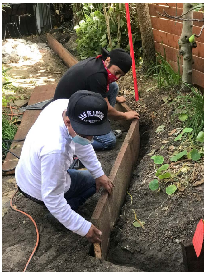
Nice mitered joints.
