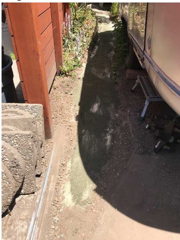
Leveled, tamped, and filled with sand and "blue fine."
