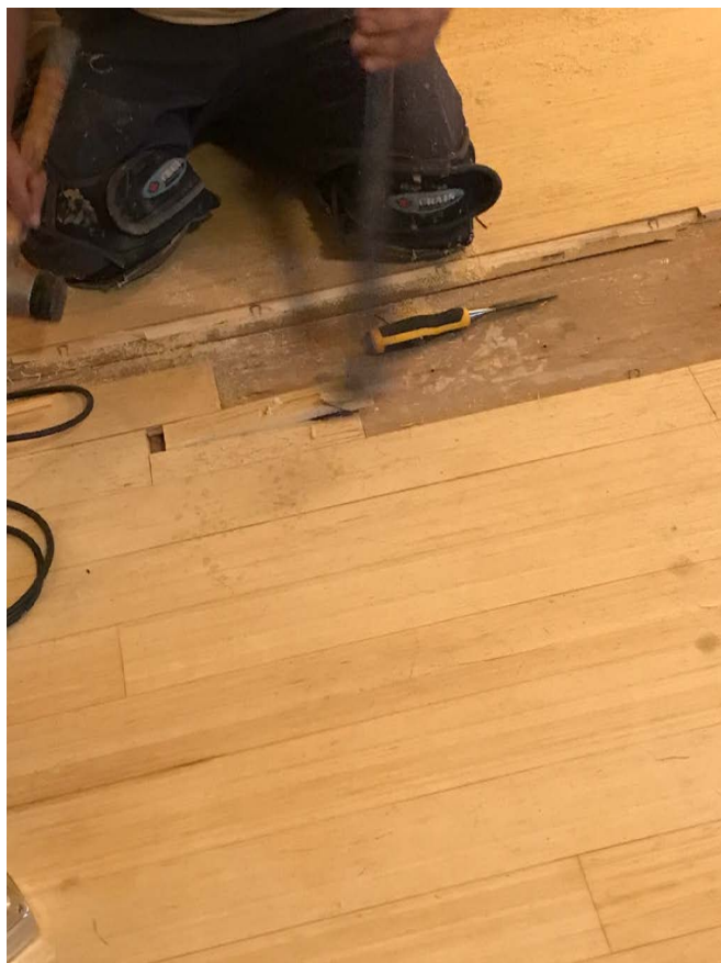
A key part of this being a better job than last time was replacing substandard boards that we put in 15 years ago. Fixed now; better late than never.
