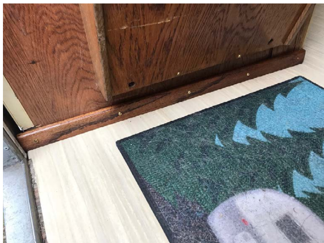
This new baseboard is stained and varnished oak with round-head brass fasteners. More to come along the bedroom wall.
