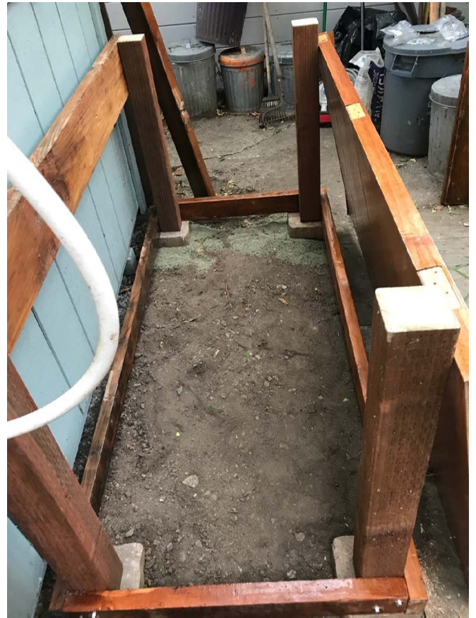
The frame is all leveled and fastened with stainless-steel lag bolts
